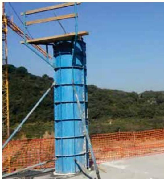
Dairesel ve Dörtgen Kolonlarda Payanda Yerleşimi (Settlement of Props at Circular and Quadrangle Columns):
